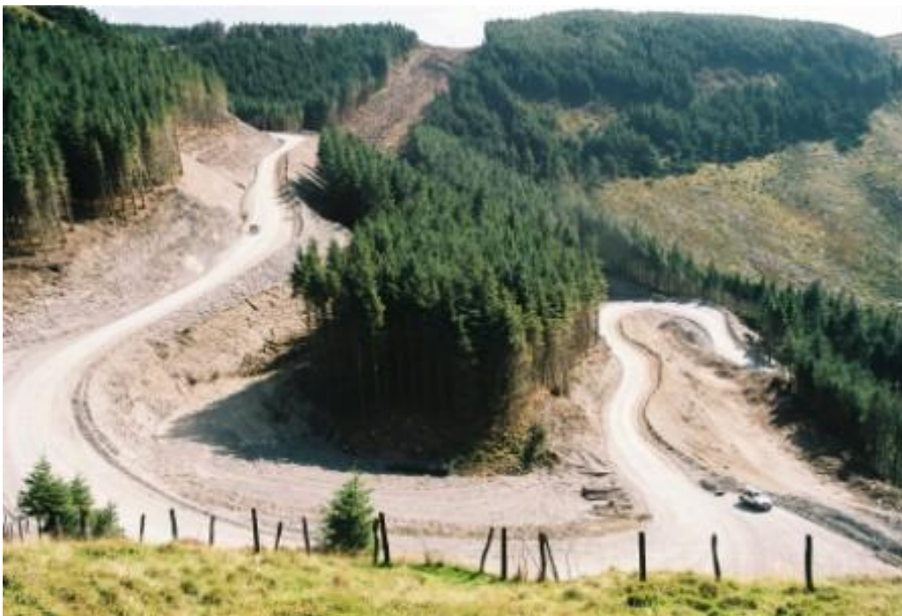
Figure 1: Windfarm access road in Cefn Croes, Wales
